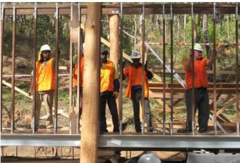
Photo: Kuku Yalanji community, ICV volunteers and EWB volunteers work together to construct composting toilets at Shipton's Flat, in the Daintree rainforest, Far North Queensland, July 2011.
